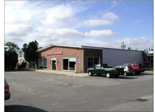
Available space seen from plaza entrance
